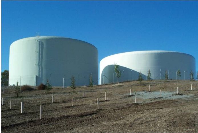
Photograph 2-2: Fairview Road Tanks
