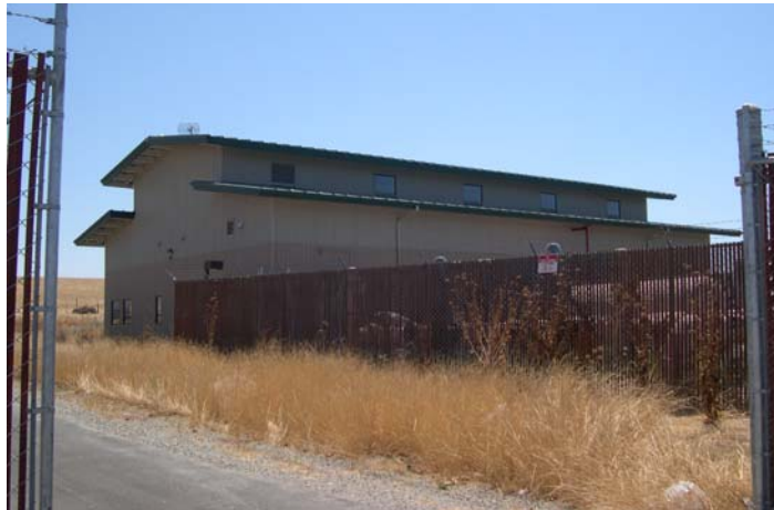
Photograph 2-1: Lessalt Water Treatment Plant
